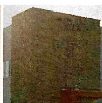
Photo 7 - Pierre Source: Google street view
